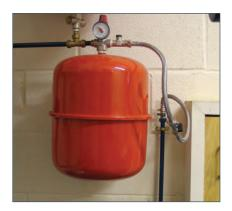
The expansion vessel and filling loop is usually positioned near the boiler.
