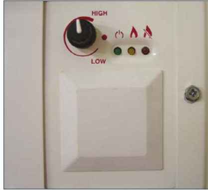
Adjust the temperature of the boiler water by turning the boiler control thermostat.
