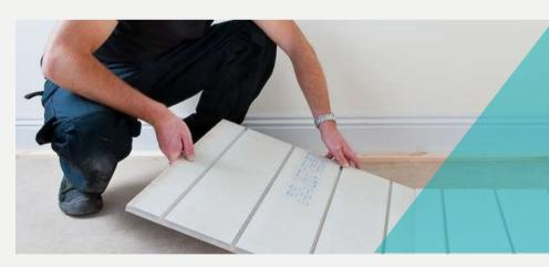
There are two main types of retrofit underfloor heating: a dry, pre-routed gypsum board that holds the heating tube; or a plastic 'egg tray' panel which is covered in a liquid compound.
